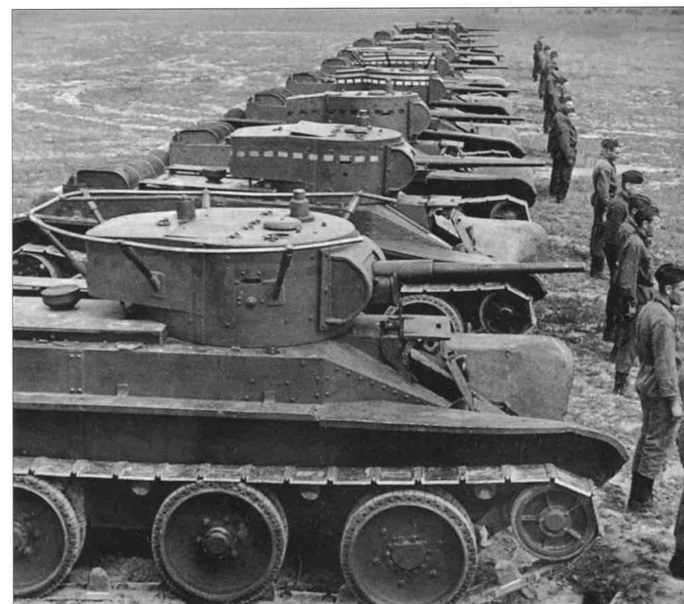
LEFT: An inspection of a Soviet BT-5 platoon; in the foreground is a BT-5U with its distinctive radio antenna. The BT-5 was effectively a BT-2 fitted with a 45mm (1.77in) gun. The original production batch had a very small rear bustle on the turret, while the production model had a more ample turret bustle. The tank went into production at the end of 1932 in a new factory in Kharkov and was the Soviet Army armoured force's backbone in the late 1930s. It had a crew of three, a new and more powerful engine, and better vision equipment. On tracks it could reach 65km/h (40mph) and on wheels a remarkable 112km/h (70mph) on roads.
